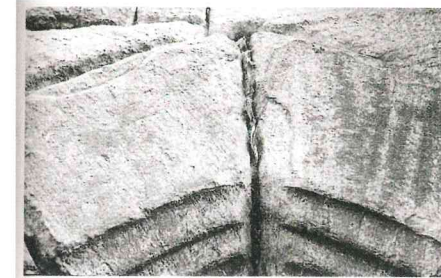
Warkworth Castle, Northumberland: oyster shells used for levelling voussoirs.
